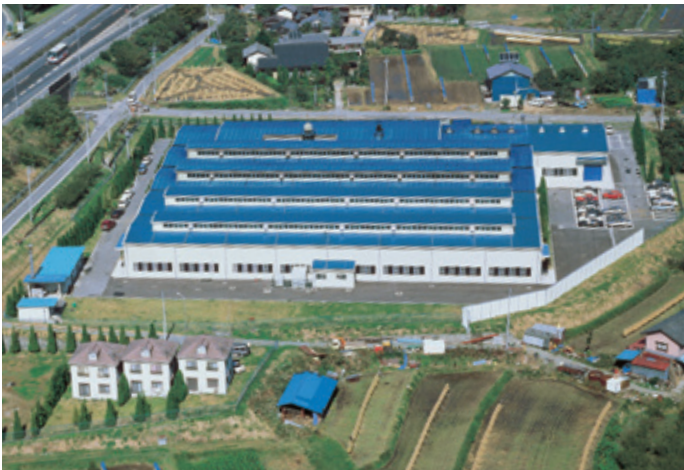
FÁBRICA IIDA - IIDA FACTORY
